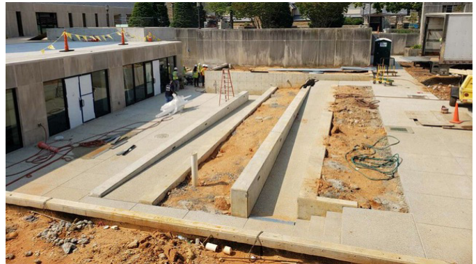
Garden terrace and ramp construction
