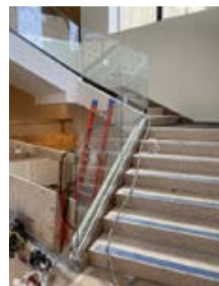
Glass walls installation.
