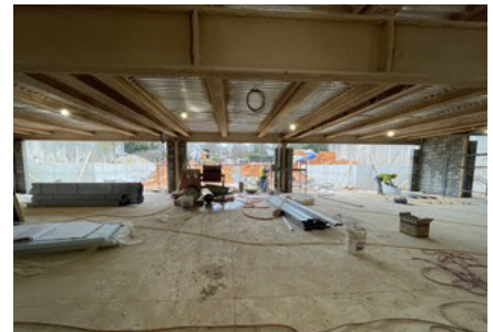
Garden Rooms taking shape
