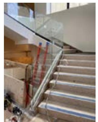
Glass walls installation.
