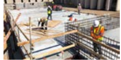
Plaza decking underway
