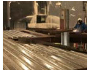
Steel for Mezzanine floor
