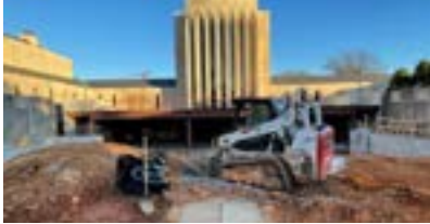
Garden Rooms progress
