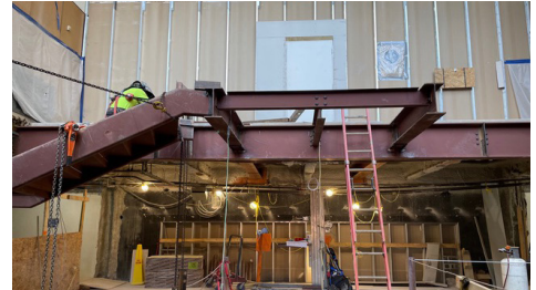
Central Stairs installation progress: Level 1 . . . . . Level 2 . . . . . Level 3!
