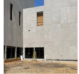
New Entrance under construction
